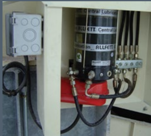
Otomatik yağlama sistemi Automatic lubrication system
