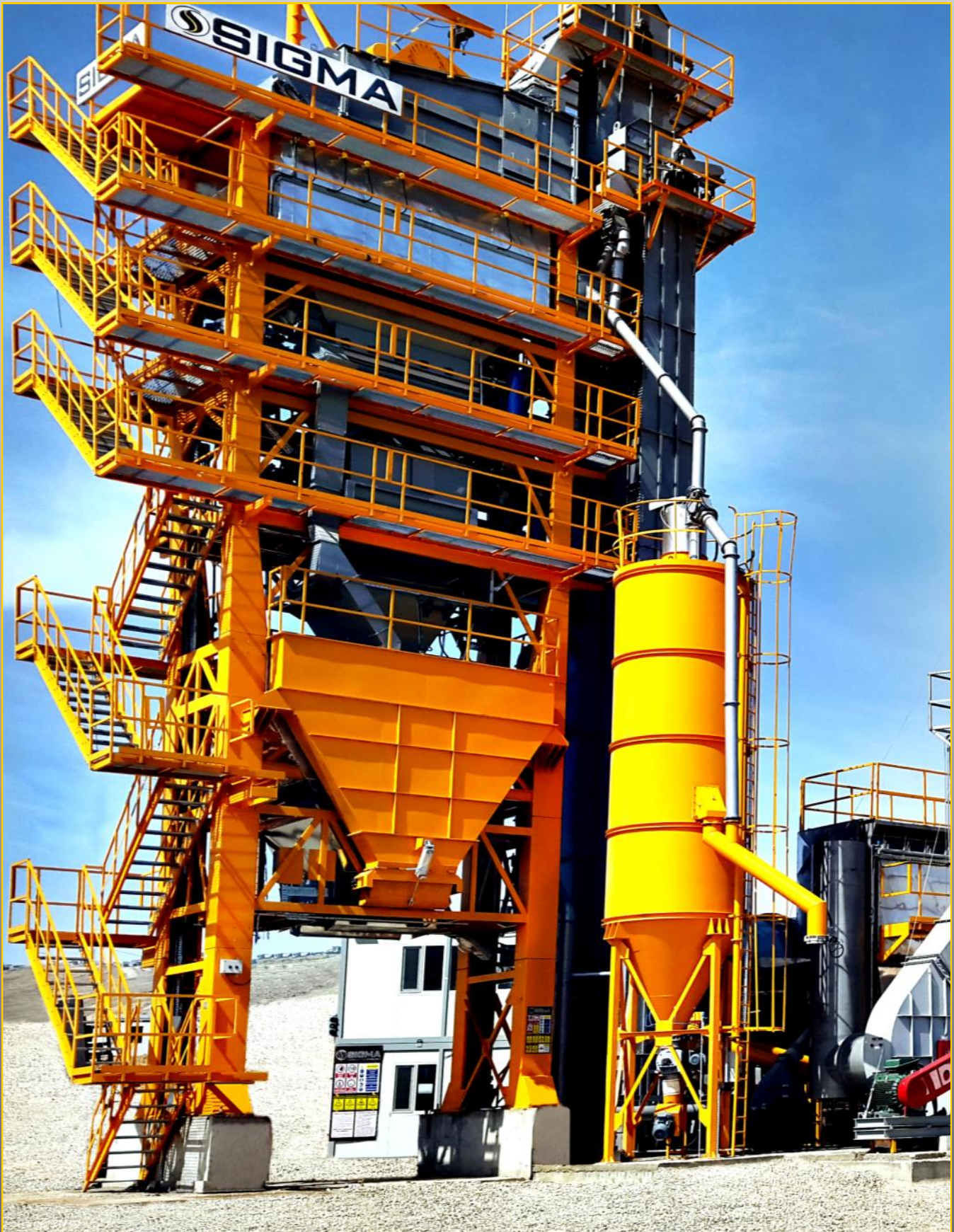
ERBIL/ IRAQ REGA ASPHALT CO. 240 T/H ASPHALT PLANT
